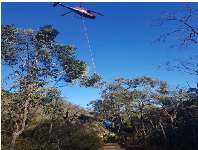
Image: Waterfall Gully Walking Trail Upgrade – Materials delivered via helicopter!
